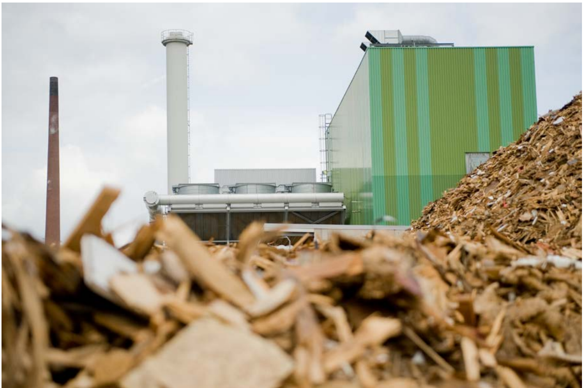
Fig. 4: Biomass CHP plant in Oberhausen
